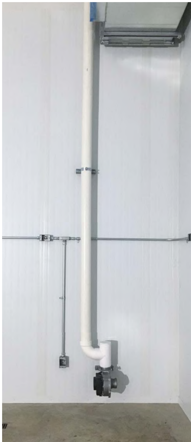
GC CO 2 Safety Valve in Dry/Cure Room
