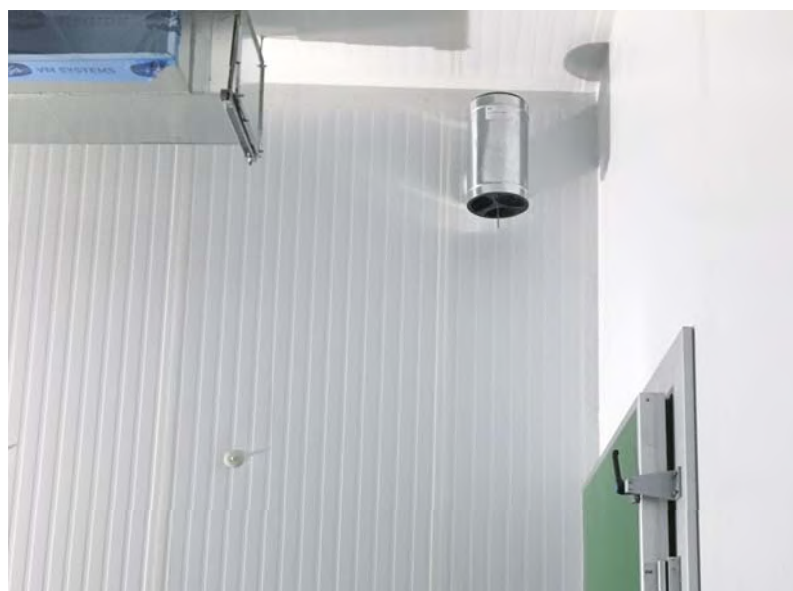
GC CO 2 Safety Valve in Dry/Cure Room
