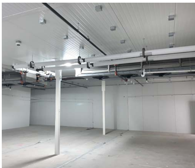
Grow Room Fit-Out with GC IMP & Refrigeration Technology
