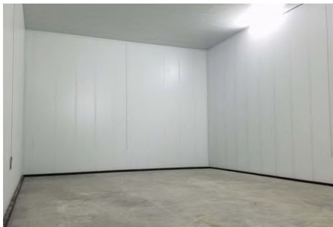
Interior of IMP CA Room w/ MPSealer & HDPE Base Board
