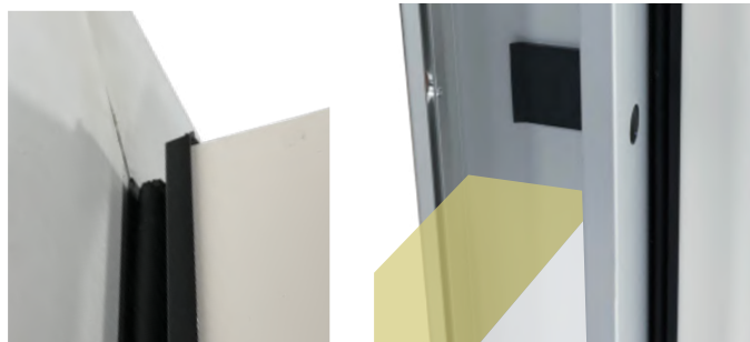
Passtight Man Door with Seal and Quick Install IMP Frame Detail
