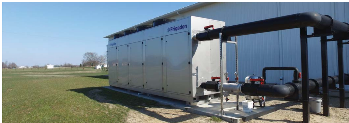
Low Profile V-Flow Dual-Discharge Coils use Less Space and Improve Airflow
