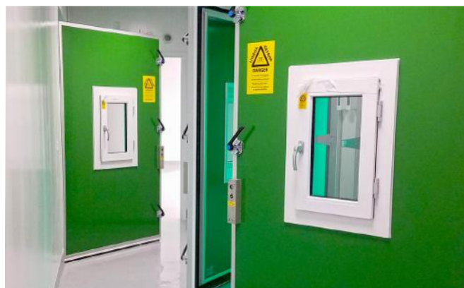
GC PA Grow Room w/ GC Gastight Doors & IMP Gastight Envelope
